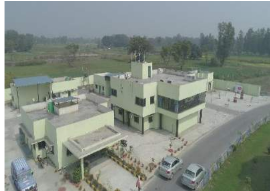
Toll Building Km. 123+490
