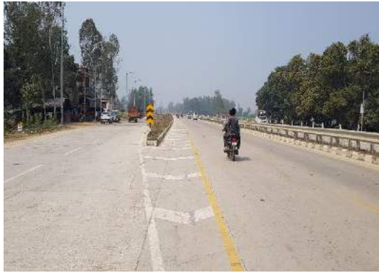
Truck Lay Bye at Km. 37+200
