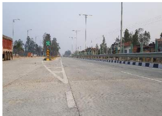
Truck Lay Bye at Km. 75+300
