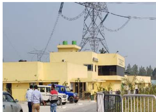
Toll Building Km. 50+900
